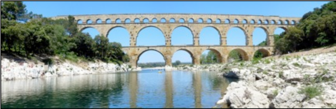
Figure 4: Pont De Gard - famous aqueduct built by the Roman Empire. The bottom level carries a road, the top level a water conduit (source: w.fr.utilisateur:Bouba )
